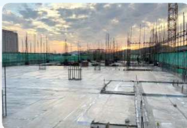
■ 项目施工现场/Project Construction Site
