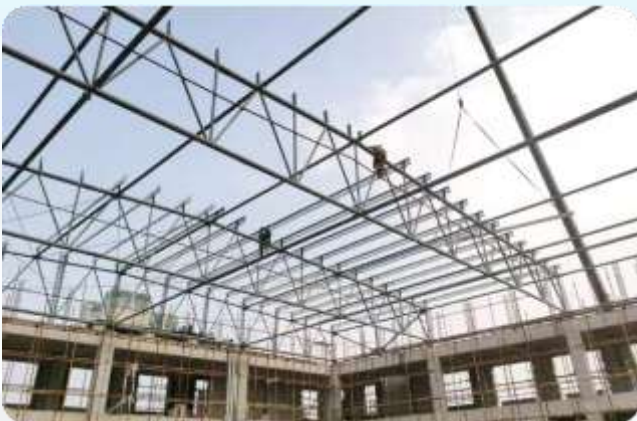
■ 保定易县小学屋面 Roof Of Yixian Elementary School In Baoding
