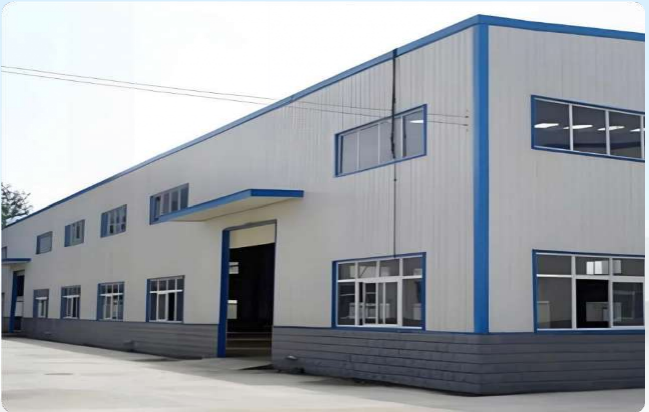
■ 华源热电厂厂房 / Huayuan Thermal Power Plant Factory Building
