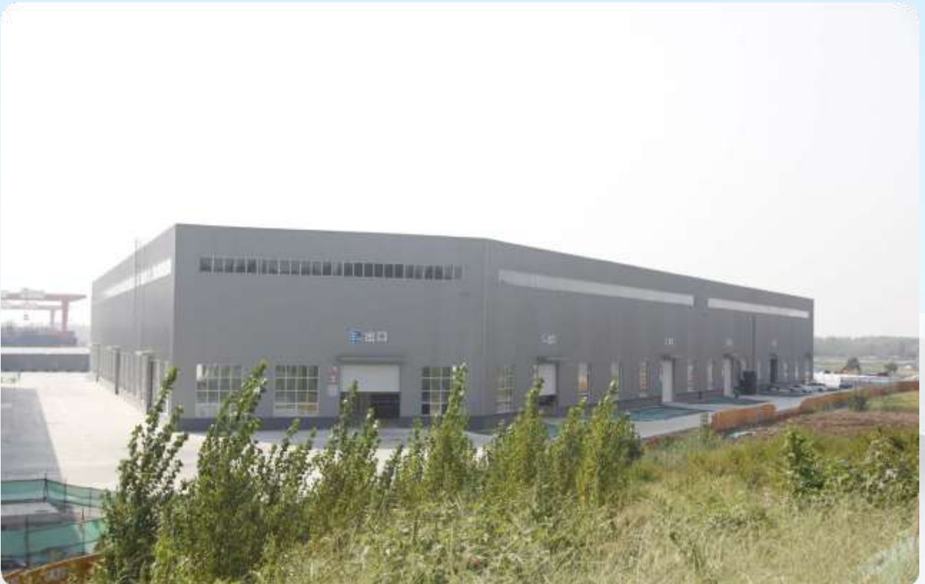
■ 龙拱港仓储 / Longgang Pofi Warehouse
