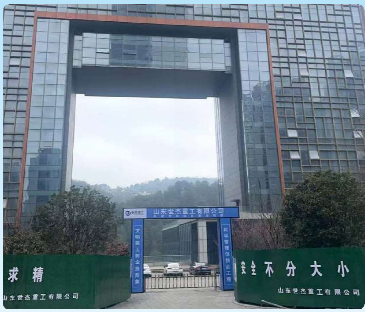
■ 贵州国宾五星级酒店装修EPC项目，21708.51平方米，客房300套，总投资20176万元 Guizhou Guobin Five-Star Hotel Decoration EPC Project, 21708.51 Square Meters, 300 Guest Rooms, Total Investment Of 20176 Million Yuan
